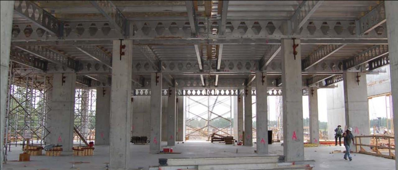
In the construction of high-rise buildings designed with long spans between columns, long bays, and repetitive floors, Patent's ROLL SHORE® system offers maximum forming productivity. Based on a grid of castellated beams and joists, the system can create and support high strength tables as large as 20,000 sq. ft. or more.
