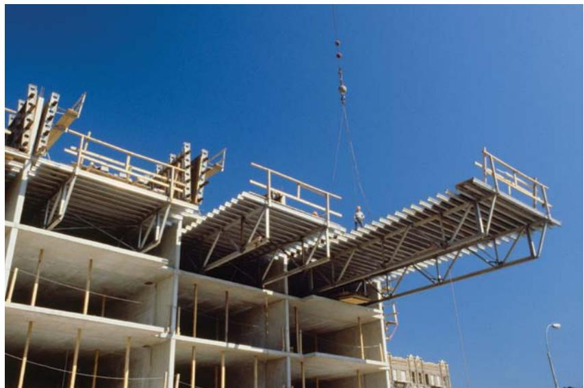
Essentially a mini-truss, Patent's spandrel beam carrier can easily be attached to the end of our 10, 20, or 30' (3.0, 6.1, 9.1 m) INTERFORM® flying tables and allows a maximum total load on each spandrel beam carrier of 10,000 lbs (4536 kg).
