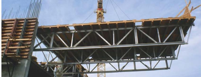
Pre-assembled truss modules are delivered to the site. Flying tables are placed into position and set to grade by adjustment of the extension legs and screw jacks. Fillers are placed in the column strips to complete the deck form.
